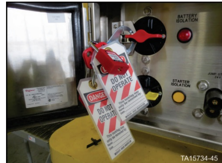
Figure 90. GEN 2 Battery Isolation Box – Battery isolation switch in OFF position with locks in place
