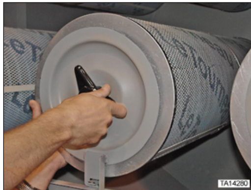
Figure 107. Installation of “KLENZ™” filter tabbed cover
