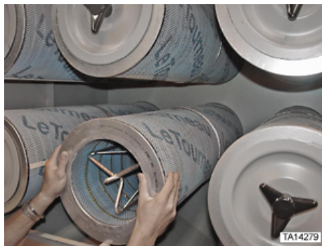
Figure 97. Removal of “KLENZ™” filters
